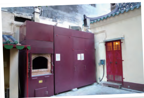
Wet-type 2-in-1 temple smoke reduction system at Hung Shing Temple, Fuk Tsun Street 福全街洪聖廟採用與濕式煙霧緩減系統二合一的化寶爐
