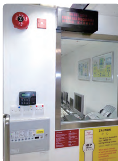
Newly Installed FM200 Gaseous Fire-fighting System 新安裝的FM200氣體滅火系統
