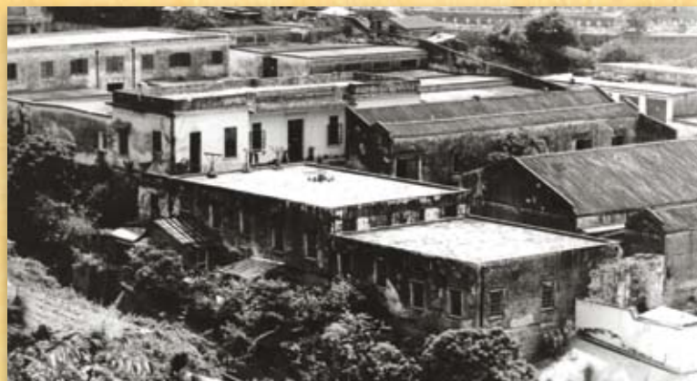
東華義莊修復前的舊貌 The old look of Tung Wah Coffin Home before restoration
