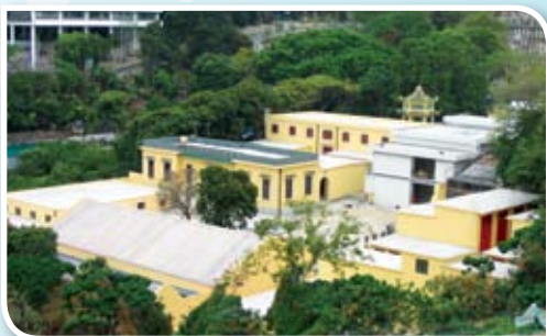
修復後的東華義莊 Tung Wah Coffin Home after restoration
