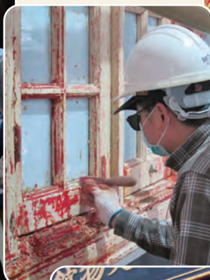
鬆漆及修復窗框 Window frame repairs
