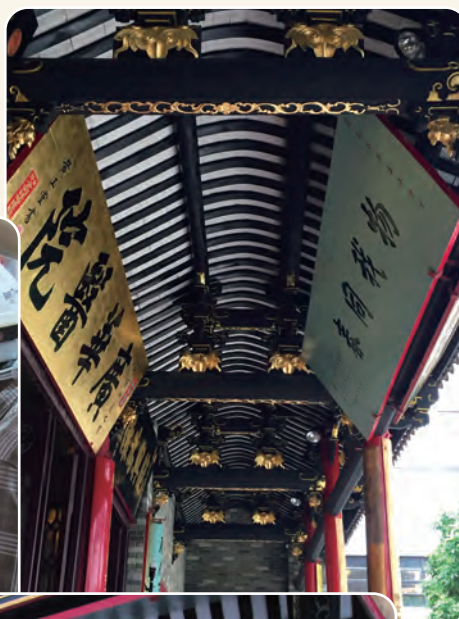
修復後的千步廊捲棚 "Humpbacked" roof at the verandah after repaired
