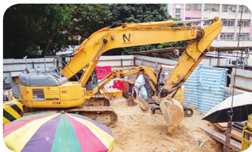
東華三院黃大仙醫院行人天橋及升降機工程經已展開。 Link Bridge and Lift Tower Project for TWGHs Wong Tai Sin Hospital is in progress.
