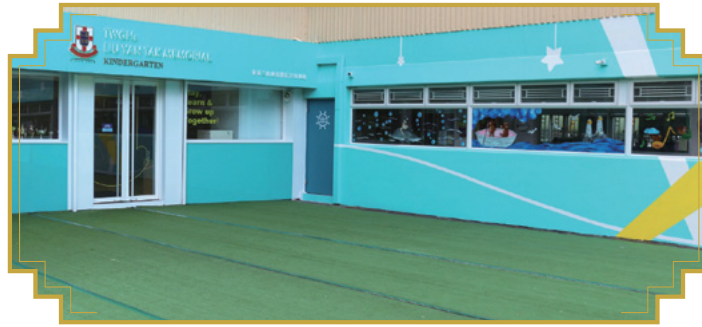
翻新後的幼稚園正門 Main entrance of the Kindergarten after the refurbishment
