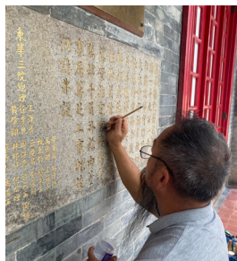
翻新文物館千步廊的紀念石碑 Restoration of the memorial stone plaque at the verandah of the Museum
